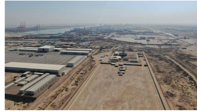
A significant milestone in the expansion of our energy assets is the construction and operation of the Umm Qasr power plant at the Basra Governorate in Iraq. The gas-fired power plant is a testament to Prime Infra's commitment to deliver critical projects and shape the socio-economic landscape of regions in need.
