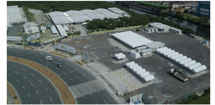
Prime Infra-led PrimeBMD supported the country's pandemic response through the construction of the first mega vaccination site that served residents from Metro Manila and nearby provinces. The vaccination site is still in operation, and has administered close to 300,000 doses as of March.
